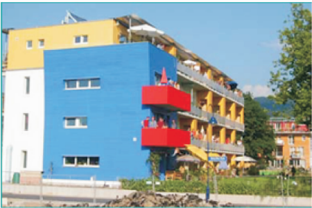
图1 2002年德国安装于住宅屋顶的太阳能真空管集热系统 Fig.1 Roof-mounted evacuated tubes at the ISIS Demonstration Building, Germany in 2002
