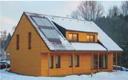
图2 2003年捷克与建筑屋顶相结合的平板式太阳能集热板 Fig.2 Roof-integrated flat-plate collectors at the House W, Czech Republic in 2003
